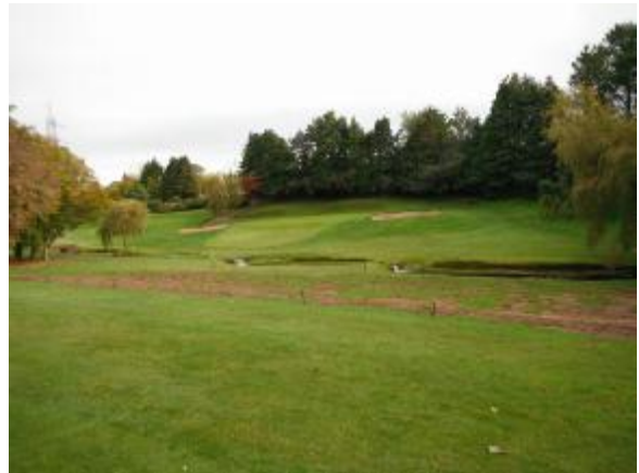
Figure 10: A main drain has been installed to the end of the 10 th fairway to capture subsurface water flow. Slit drains may be needed in time to intercept surface water from higher ground.
